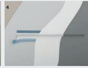
Apply two or three coats of plaster.Apply the gauze over the joints.Sand and paint.
